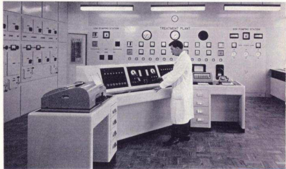
The Control Room
