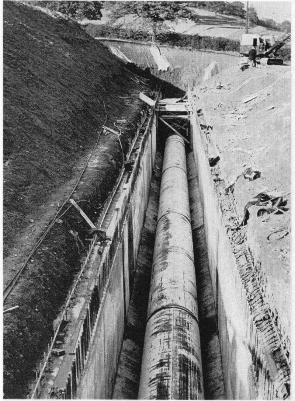
Diversion Culvert and Outlet Main – construction stage
